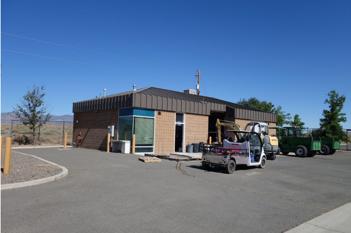
Maintenance Shop - Building #2500 Description: Exterior of the Building.
