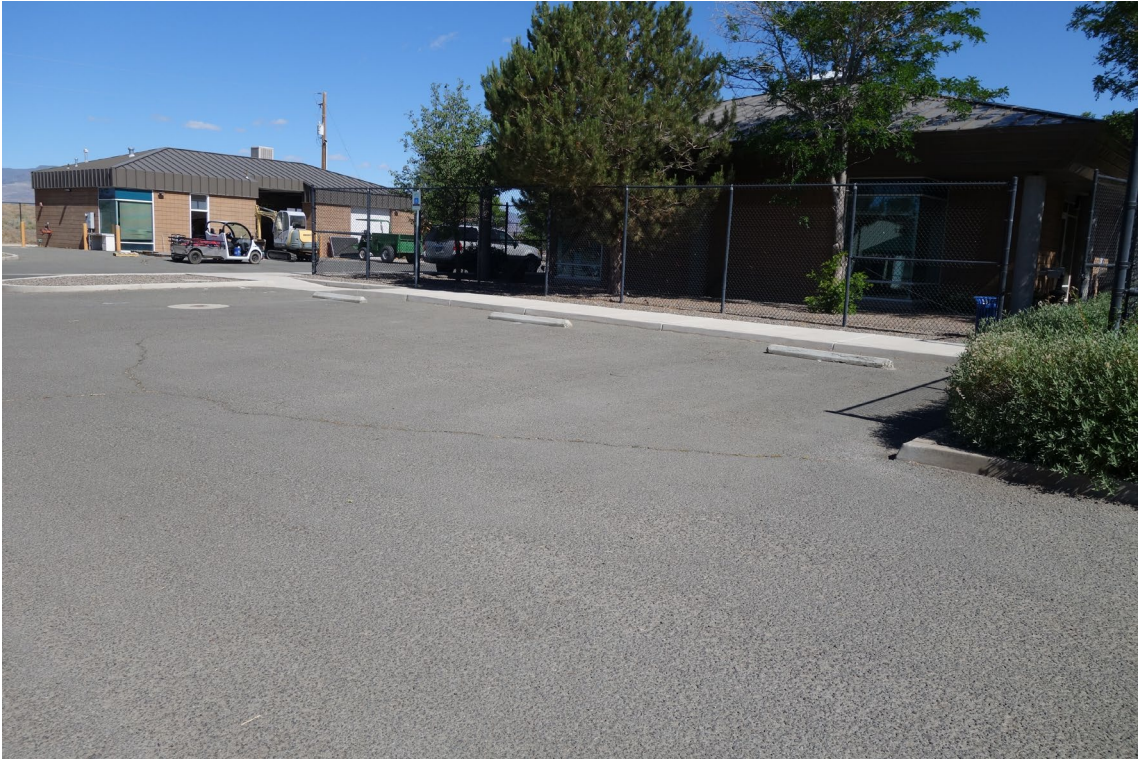
Northern Nevada Veterans Memorial Cemetery Site - Site #9898 Description: Slurry Seal Paving Project.
