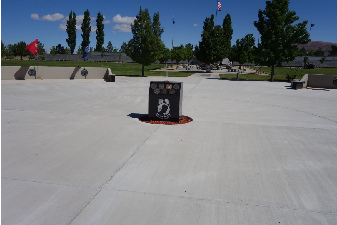
Northern Nevada Veterans Memorial Cemetery Site - Site #9898 Description: Concrete Courtyard between the Pavilion and Public Information Building.
