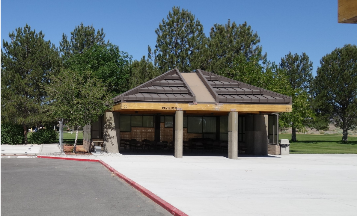
Cemetery Pavilion - Building #1943 Description: Exterior of the Building.
