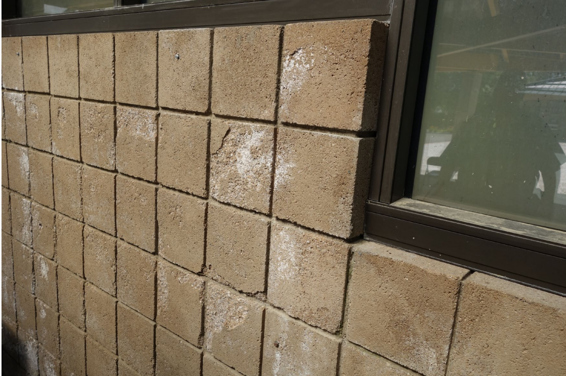
Cemetery Pavilion - Building #1943 Description: CMU Decorative Block Replacement Project.
