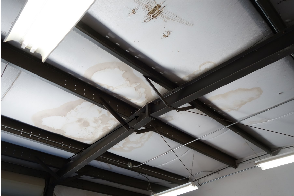
Cemetery Welding / Storage Shop - Building #1942 Description: Roof Replacement Project – Multiple Roof Leaks.
