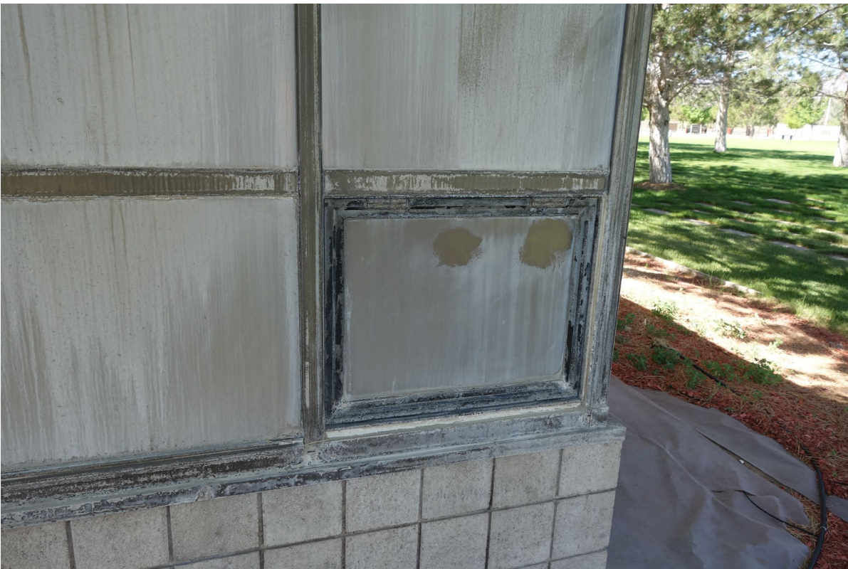
Cemetery Pavilion - Building #1943 Description: Glazing Replacement Project.
