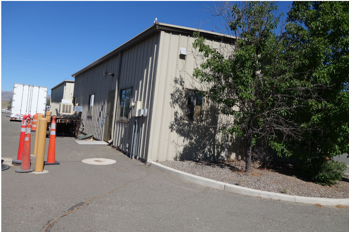
Cemetery Welding / Storage Shop - Building #1942 Description: Rear Exterior of the Building.
