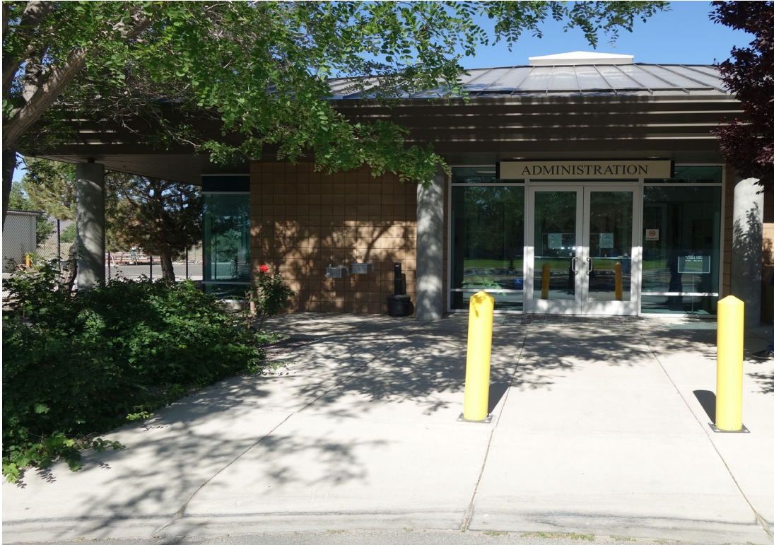
Administration Office - Building #2499 Description: Exterior of the Building.
