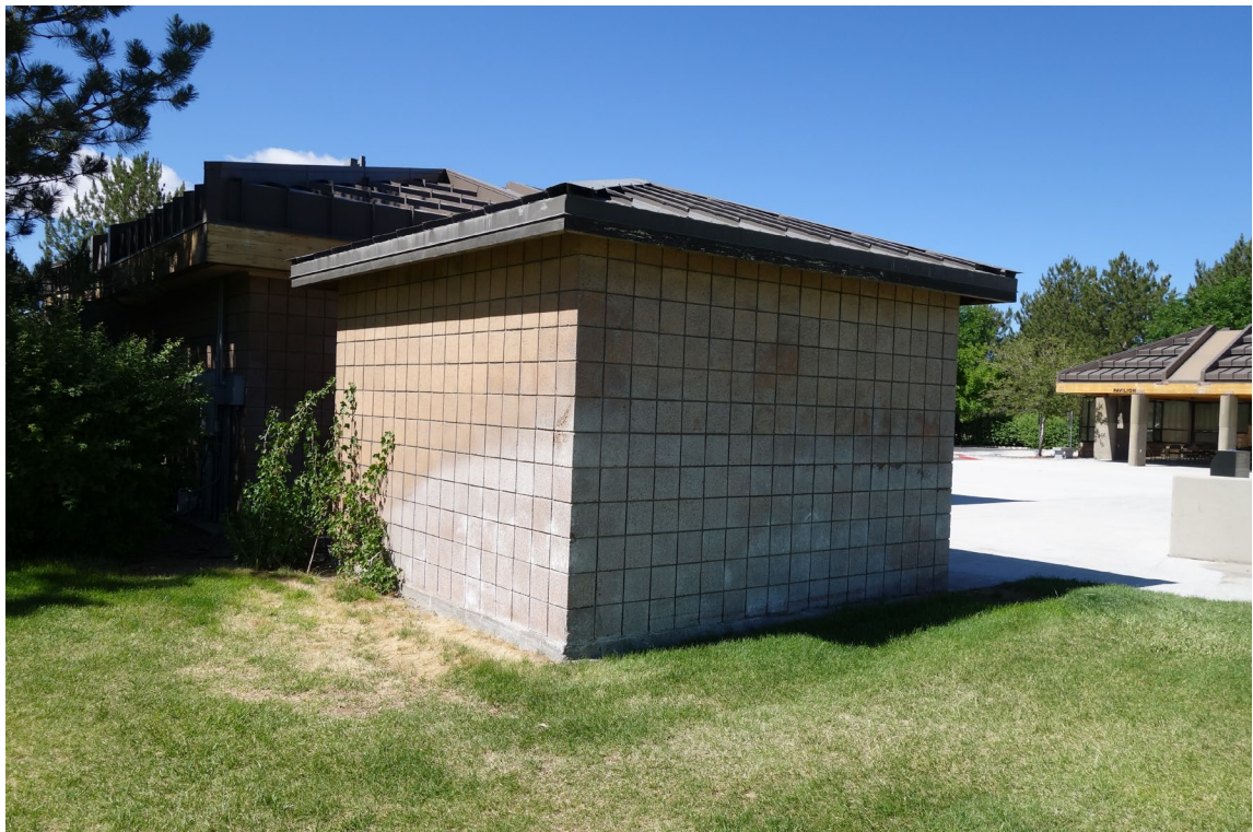
Cemetery Storage 2 - Building #2036 Description: Exterior Finishes of the Building.
